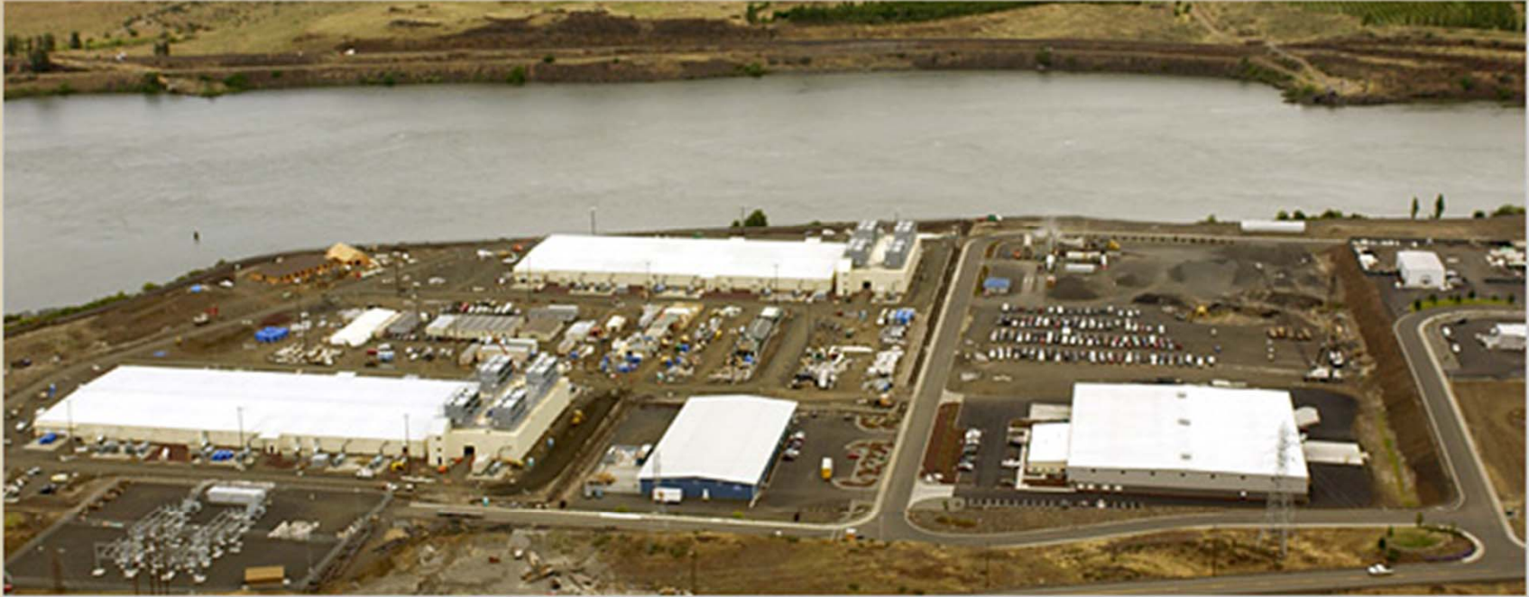
Google Data Center on the Columbia River in Oregon.
